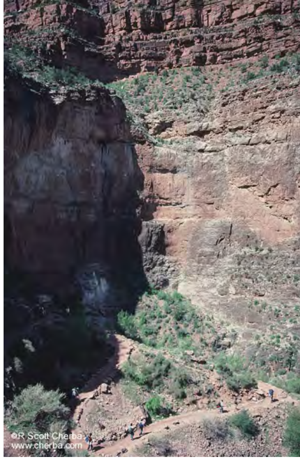
Redwall Limestone along the Bright Angel Trail. Note vertical streaks and rock spalls.
